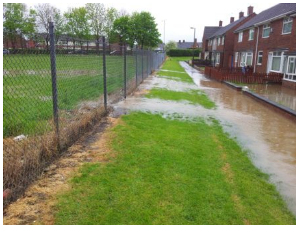
Photograph 2 – Clearly shows the source of flooding as run off from the Arqiva site, the water is collecting at the low point and flooding properties
