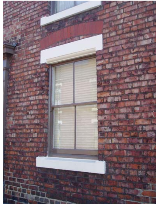
Typical 4-pane window with arch detail
