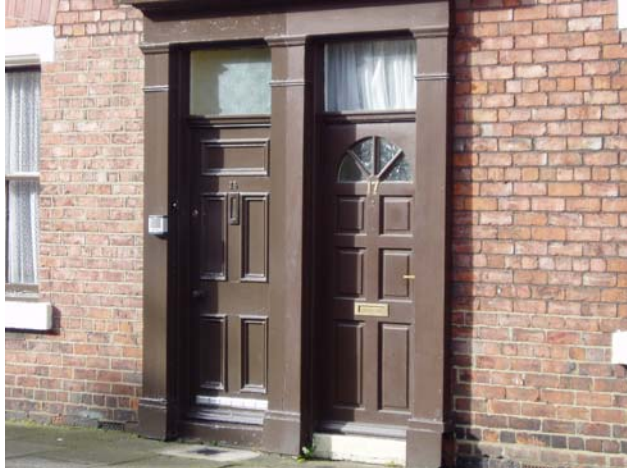
Original colour, but the door on the right is modern and of the wrong design for this period.
