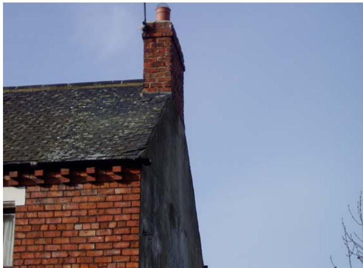
Ornate eaves detail and tall chimney
