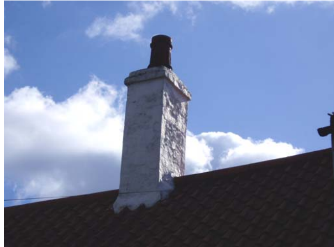
Large slender chimneys are attractive
