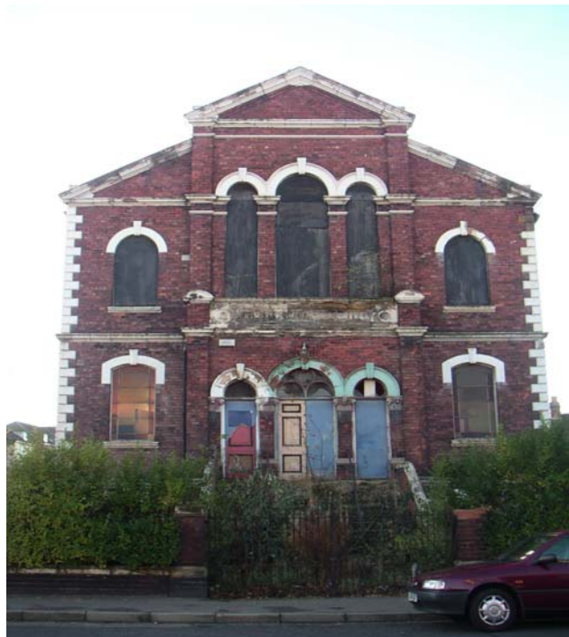
Buildings such as this Victorian Primitive Methodist Chapel required a full historic survey prior to demolition.
