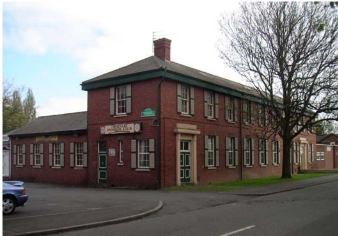
The Former Drill Hall at Thornaby Aerodrome.
