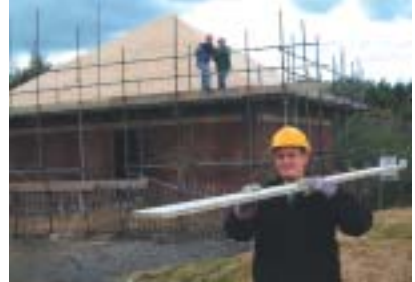
Planetarium under construction
