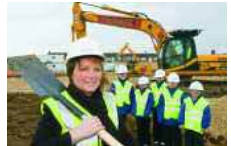
Headteacher Ruth Pickering and pupils of Hardwick Primary School set work on their new school under way.
