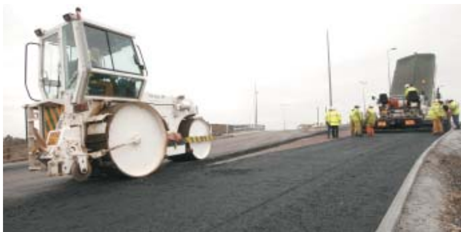
Contractors put the finishing touches to South Stockton Link
